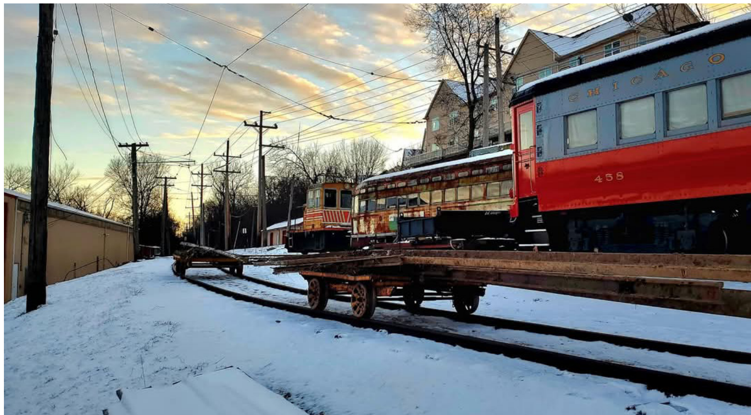
Fox Valley Trolley Museum volunteers have been using small flat cars to move rail so they can save as much money as possible in building an addition to their storage barn, officials said. ERIC ZABELNY
